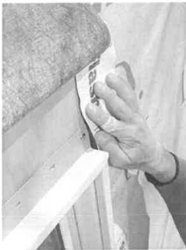
1. Lap The Flashing Tape
