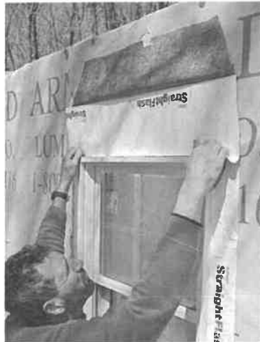
2. Run The Tape Over The Jamb
