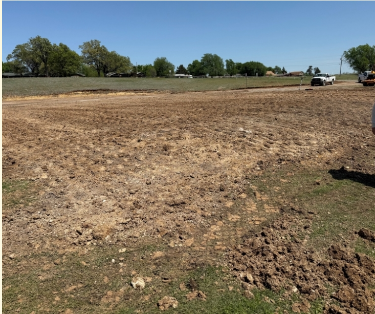
New leveled land for dry stall installation (above)
